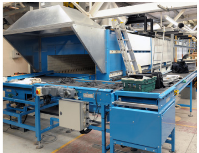
Pictured: New kiln currently being installed in our Stoke-on-Trent factory.
